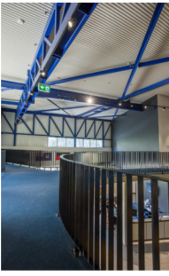
BALUSTRADE DETAIL - IN NATURAL GALVANISED STEEL
